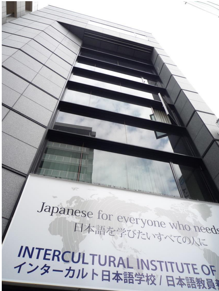
7階建て校舎 Seven-story school building
