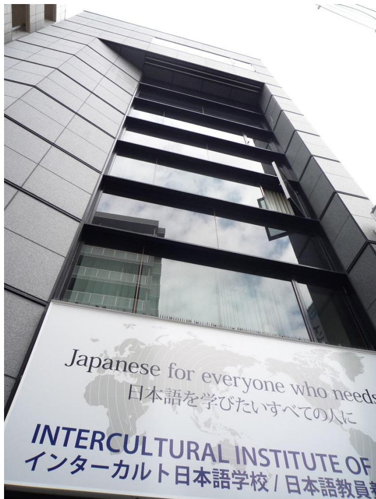
7 階建て校舎 Seven-story school building
